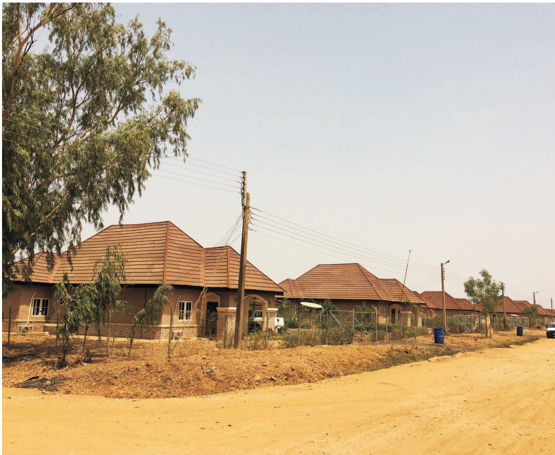
Rehabilitated Savannah Sugar Staff Housing Estate
