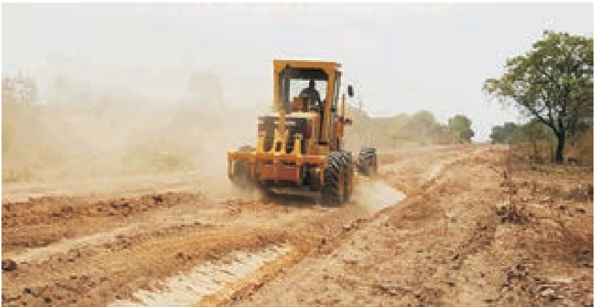
■ Land preparation activities @ Tunga Sugar Project Site
